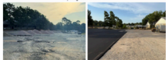
Paving project is in progress from Close Hatches to Vandalingham.
