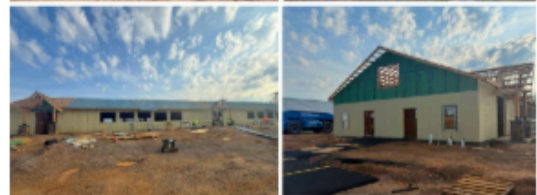
Construction is underway on the new 28-stall barn.
